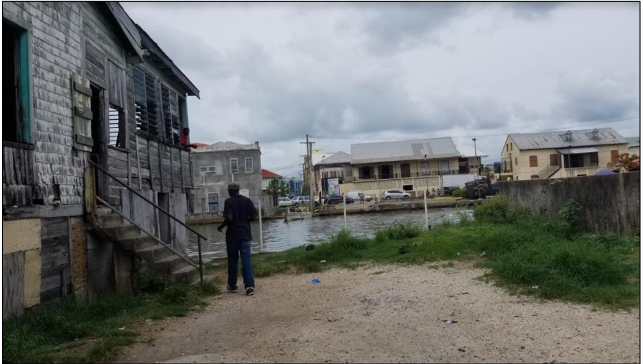
Image 1: Bar (on left) bordering the canal in the back. Non-elevated businesses in this area reported intense flooding inside their businesses during times of high-tide.
