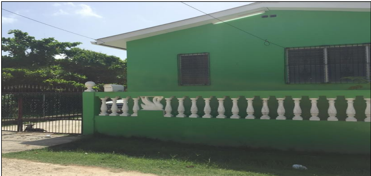
Image 10: Jane Usher plot 175 (N 17.48487 W 088.20587) is a homemade of masonry, which is the most resistant to flooding and hurricane damage.
