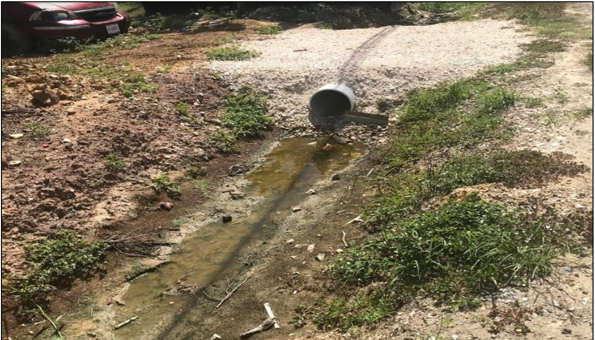
Image 7: (N 17.48462, W 088.20471) A drain on plot 131 on Jane Usher Boulevard harbors standing water due to inefficient drain construction, leaving a breeding ground for mosquitoes.
